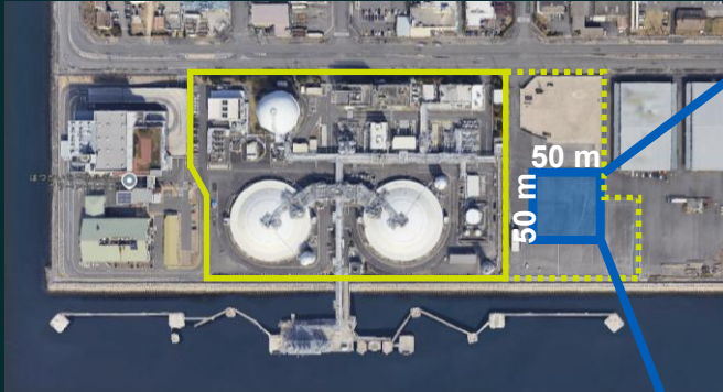
Hiroshima Gas Co., Ltd. Hatsukaichi Plant
