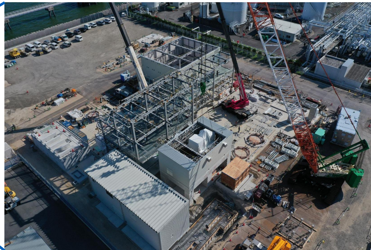
Image of construction site
